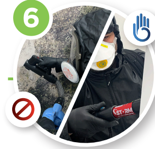
6 A. Spray any visible mould with FloodHit and wipe down. B. Apply BioTouch.
